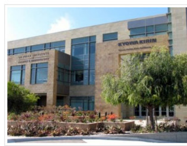
The exterior of the LJIA facility. Photo: Courtesy
