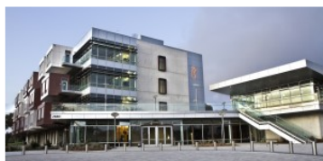
The new headquarters for the Sanford Consortium for Regenerative Medicine. Courtesy Sanford Consortium.
